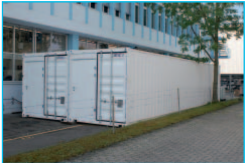
Typical containerised ozone generation systems
