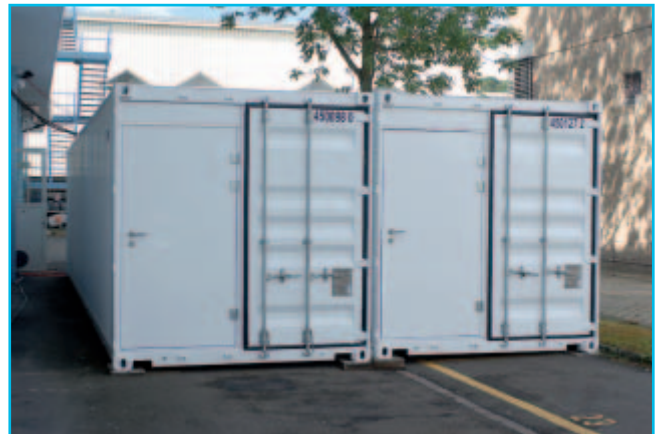
Complete plant seen from the outside
